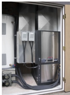
Typical Residential Geothermal System
