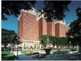
Chicago Hilton and Towers
