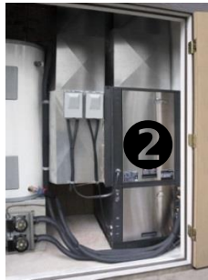
Typical Residential Geothermal System
