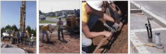
Geothermal Loop Installation
